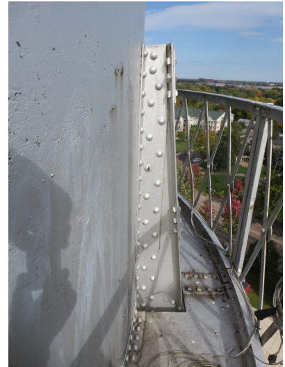
Riveted connection of tower leg to the tank.
