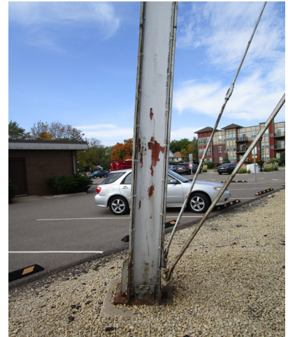
Peeling paint on southwest tower leg.
