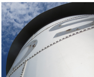
Paint damage on the tank exterior.
