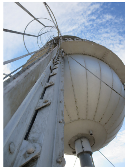
View of the cage ladder on the northeast leg of the tower and the hemispherical tank bottom.
