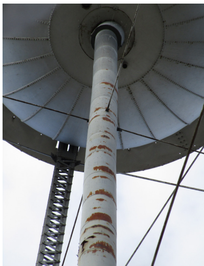
Photograph of riser shaft showing the corroded steel and the insufficient joint between the shaft and the tank.
