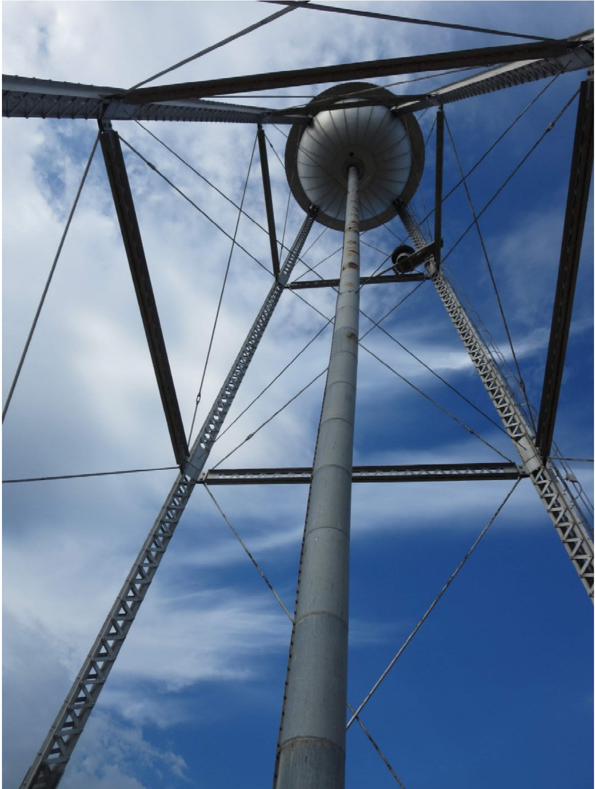
Photo 15 - Base of tank and bracing - note dark spots on bracing are surface rust locations
