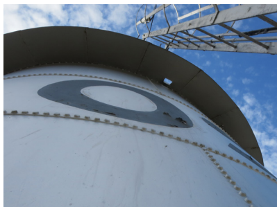
Flaking paint on the "O" on the north side of the tower.
