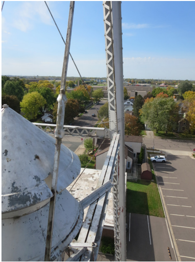
Close up view of emergency siren at northeast corner of the water tower.
