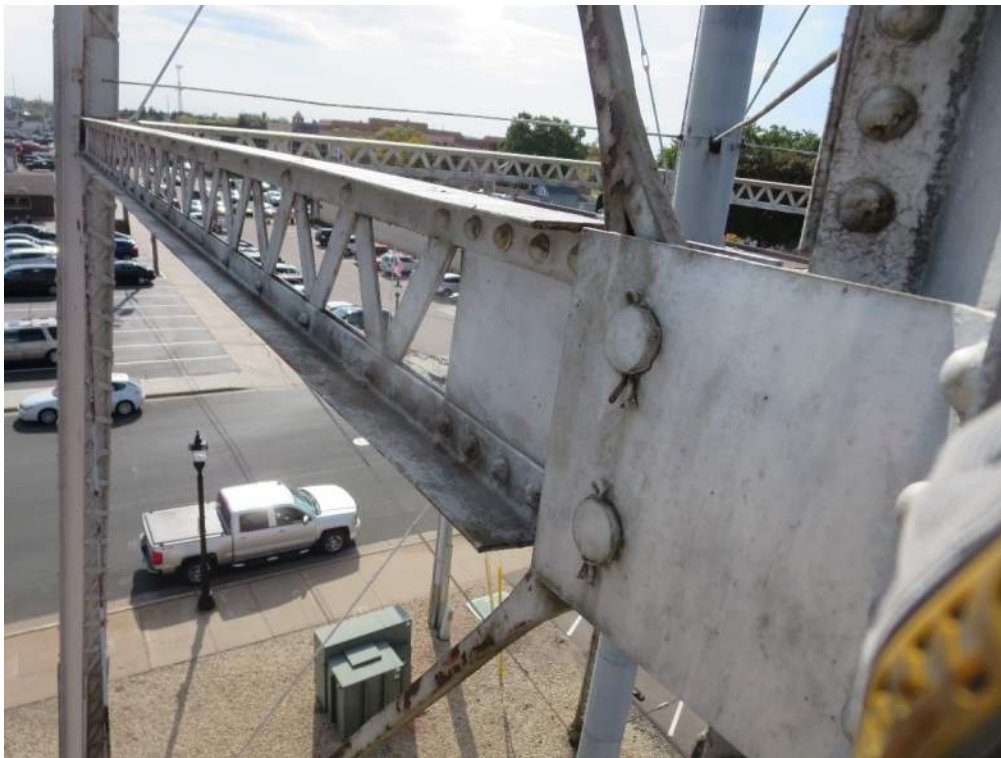
Photo 7 - Horizontal beam - note: cotter pins intact
