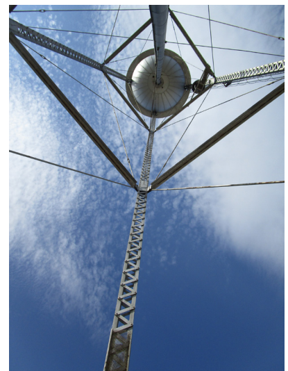
Photograph of the hemispherical bottom, taken from the ground near the standpipe.
