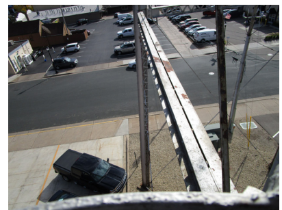
Peeling paint on structure, photograph facing south.
