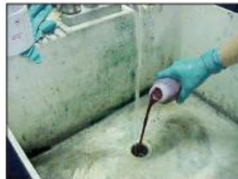
**Figure 63: Dye Testing Plumbing (NEIWPCC, 2003)**
